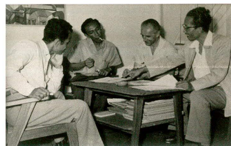
Ries Mulder in a workmeeting including Ahmad Sadali, 1950s.
