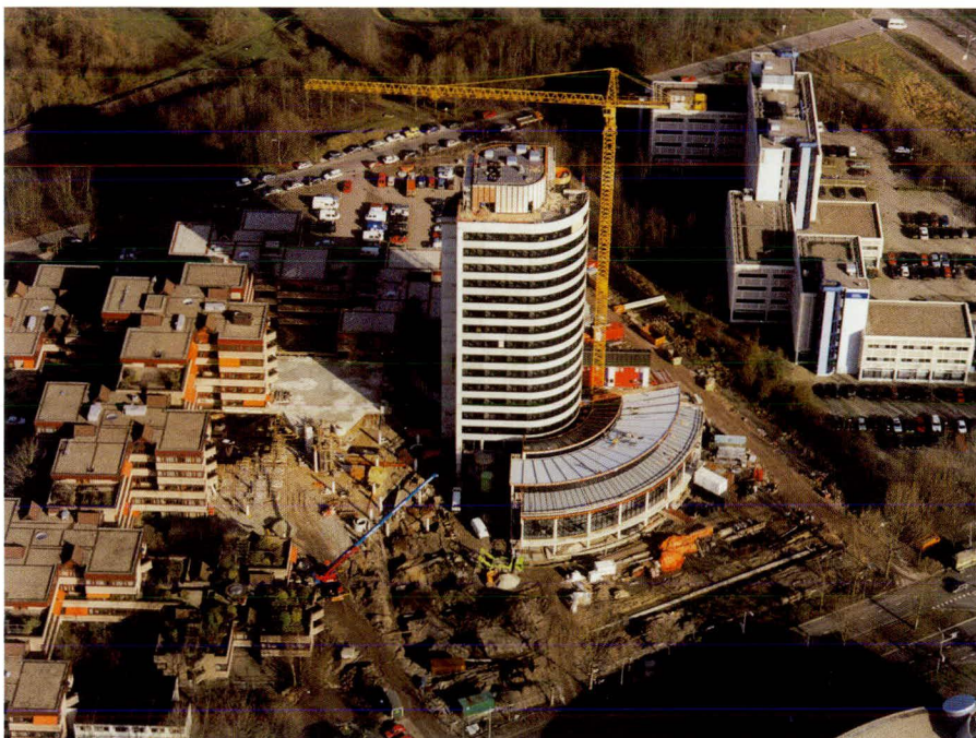
The new provincial buildings in Rijnsweerd under construction, 1995.
